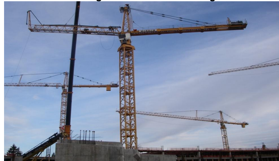
Erection of Tower Crane #4
