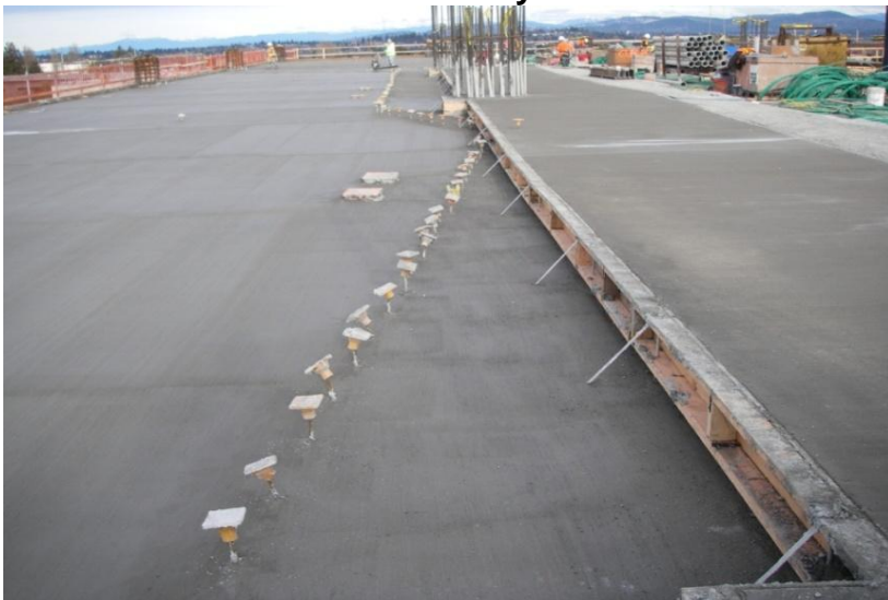
RCF building: 5 th floor @ NW corner
